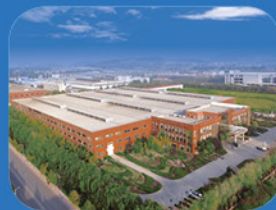
Laishan Industrial Park
